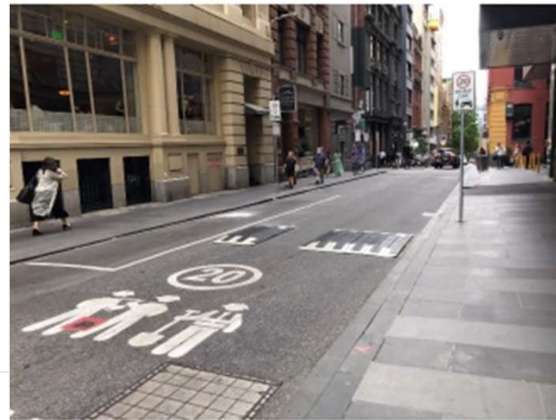
Mid-block repeater treatments of speed cushions and stencils
